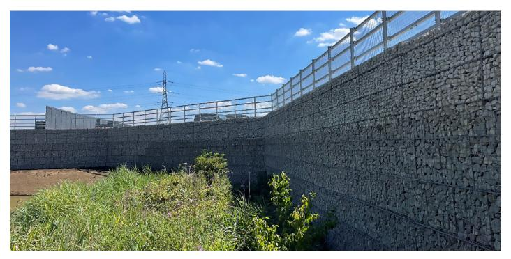
**Project Scope:** The project scope encompassed the installation of gabion cladding on both sides of the First Bait Bridge. Gabion baskets, supplied by Hy-Ten, were strategically placed to cover the existing grey concrete walls.
