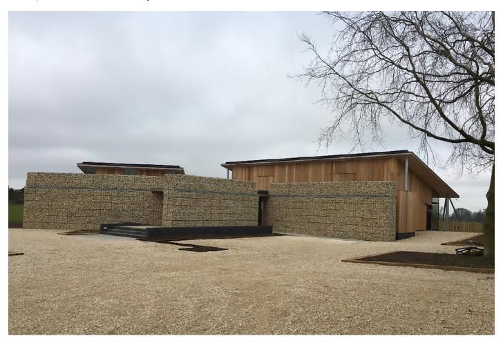
**Gabion Cladding Selection:** Western Red Cedar and Limestone-filled gabions were chosen as the primary materials for the building's external cladding. This selection was made to ensure that the structure blended harmoniously with its rural surroundings. The combination of these materials created a unique aesthetic, marrying rustic and contemporary elements.
