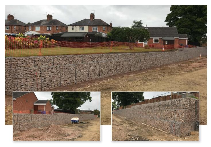
Hy-ten designed and manufactured the gabion units using Triple life coated 76.2mm x 76.2mm welded mesh in 5.0mm wire diameter.
